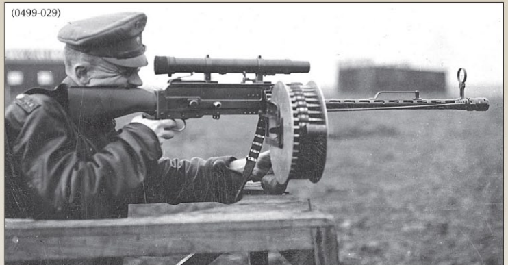
LMG 14/17 Parabellum machine gun carried by late production AEG G.IV during 1918. The Oigee sight (G5) was of limited to no use at night and was not usually fitted.
